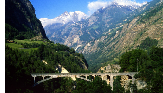
Structural and Slope Monitoring
